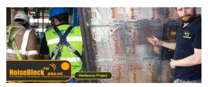
NoiseBlock BBB-DS6 material has been used successfully at Singapore MediaCorp Mediapolis mitigating 30,000.00 square meters of coverage as an integral part of their noise control mitigation measures for their newest built broadcasting and television studios production facility. The system was designed as a replacement to transitional noise mitigation cladding works which saved over 1 million Singapore Dollars for the client compared to traditional methods.
